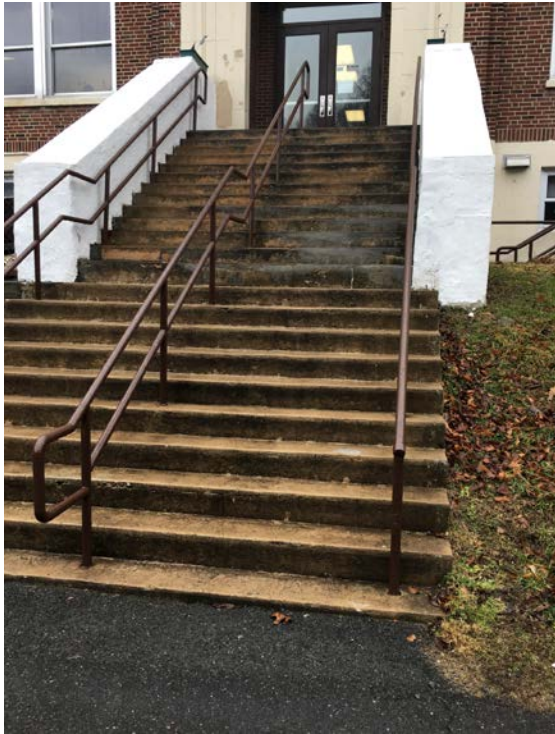
Main entry stairs and rails
