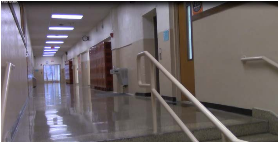
Upper floor classroom corridor
