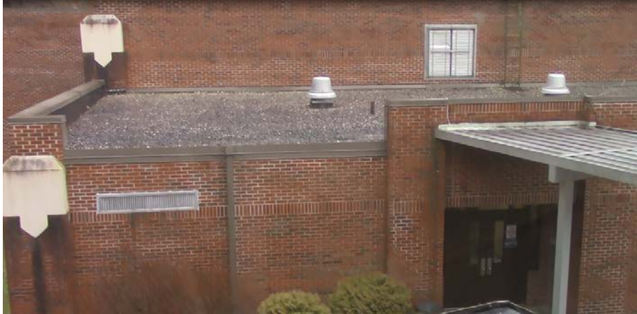
Gym building roof
