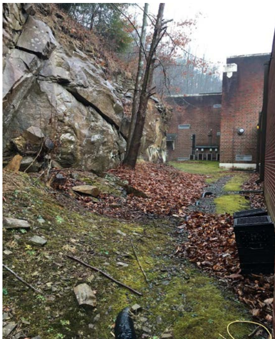
Rear of building/downspouts
