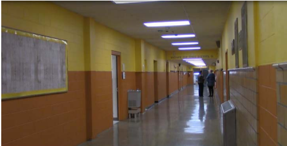
Main floor corridor
