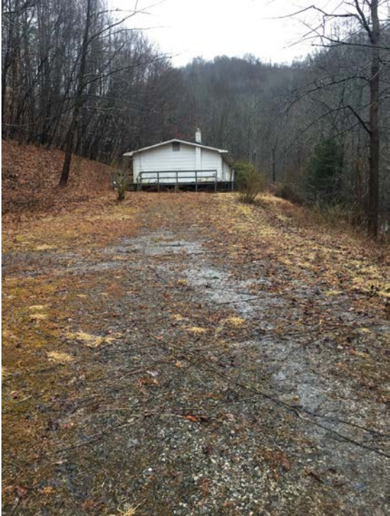
Janitors house and gravel drive
