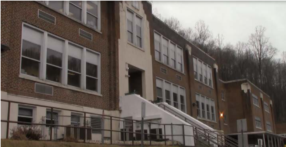
Front of original building and 1967 addition
